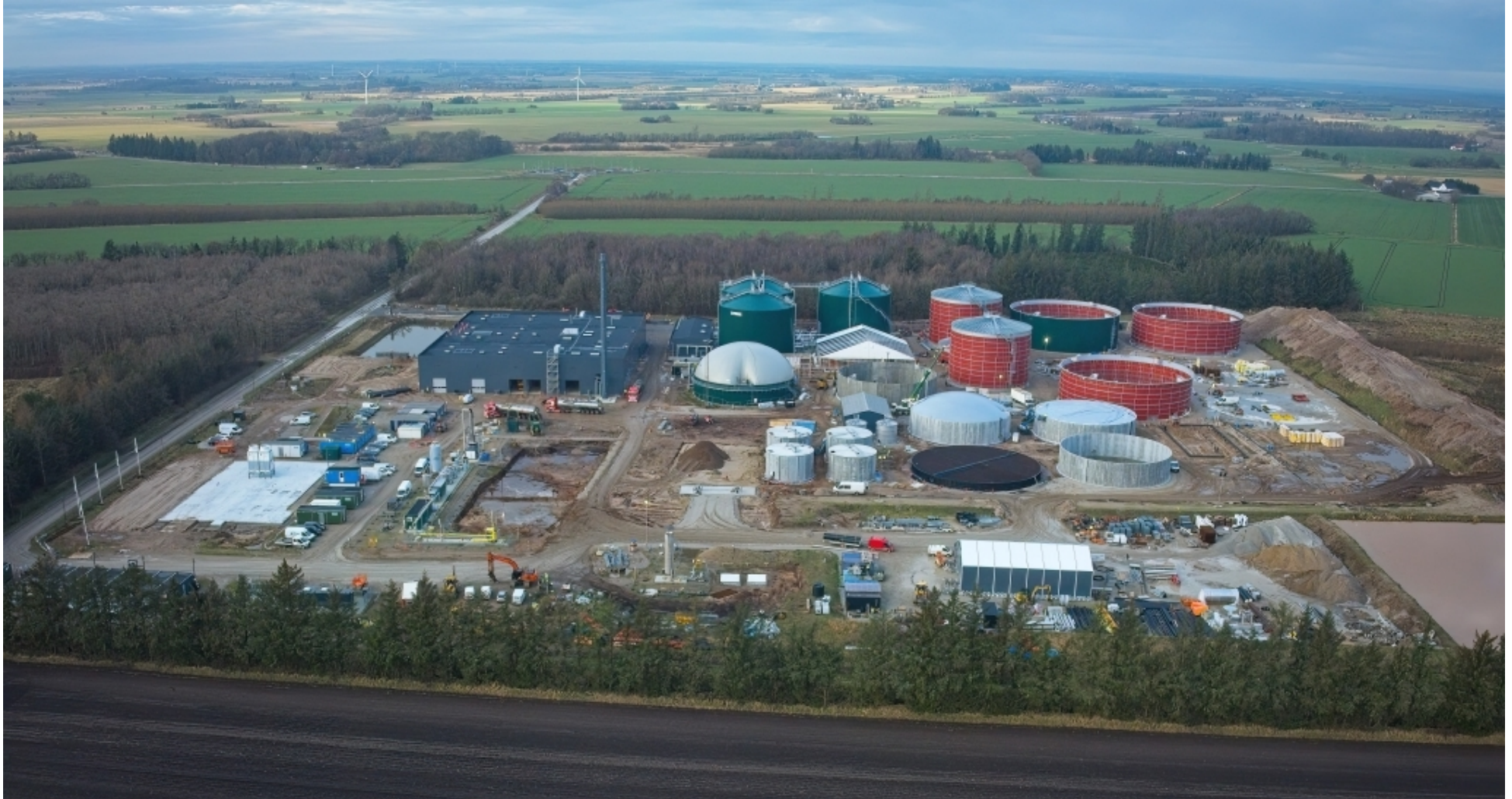
Tønder Biogas site overview, December 2023
