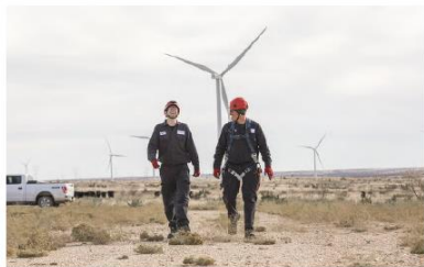
Amazon Wind Farm, Scurry County, Texas, the US.
