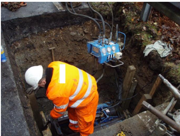
Pitmaskine under installation
