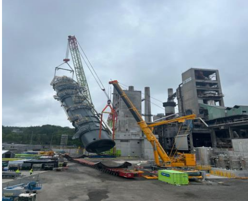
Norcem, Cement, storage
