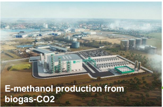
E-methanol production from biogas-CO2 European Energy, LEGO, Novo Kassø, near Aabenraa, Denmark 32.000 tons/year (2024) – to be used for POM plastic
