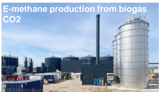
E-methane production from biogas CO2 Nature Energy, Biogasclean, Andel, SDU Glansager, near Sønderborg, Denmark 4 million m3/year (2023), 13 million m3/year (2024)
