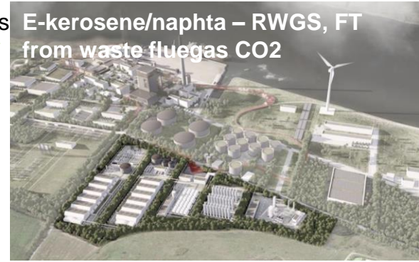
E-kerosene/naphta – RWGS, FT from waste fluegas CO2 Copenhagen Infrastructure Partners, Reno Nord, Aalborg Forsyning, Aalborg, Denmark 80.000 tons e-kerosene/y + 17.000 e-naphta/y (2027)
